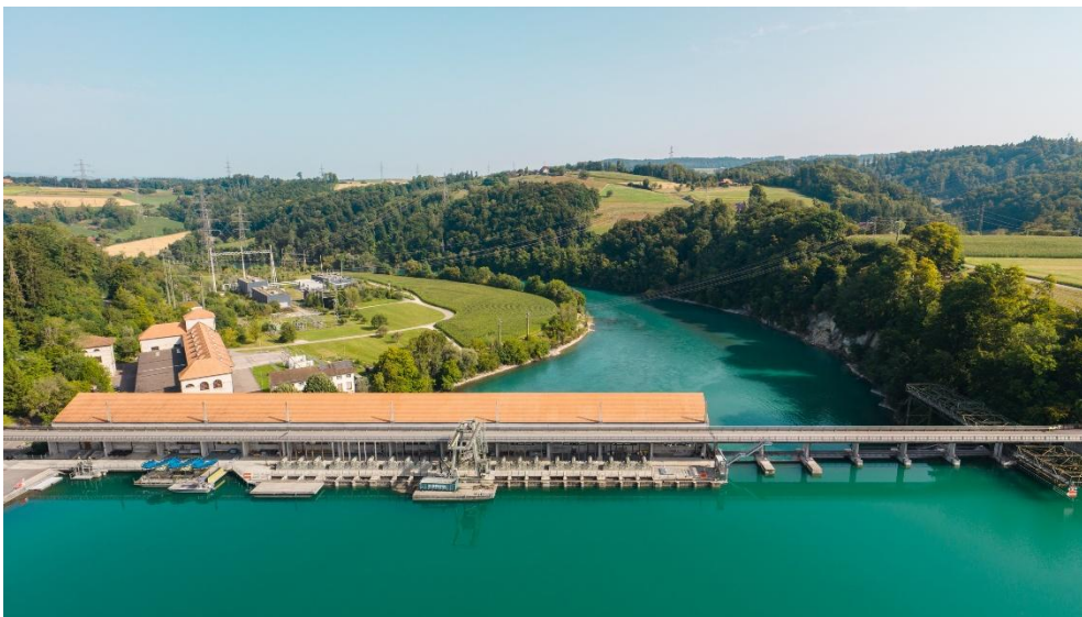
The Mühleberg hydropower plant and substation (© BKW, Daniel Hager)
